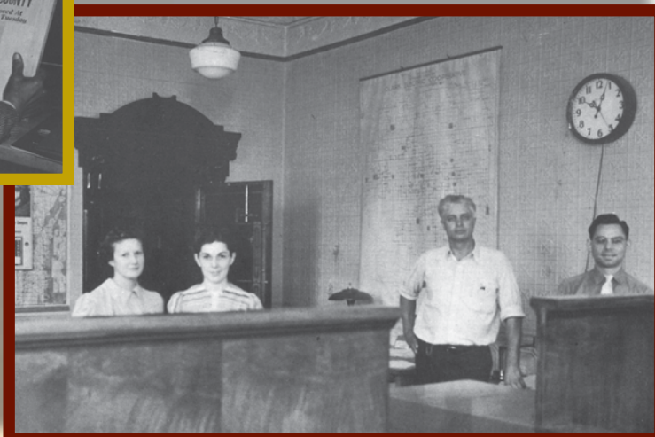
In 1937, office quarters were rented in the Hoehne Building in Greenwood to give first visible evidence that Clark Electric Cooperative was an established business. In August 1940, when this picture was taken, the office staff had grown to four. Left to right are Sylvania Kokley, Marie Kunce, Manager William Dallman, and Bookkeeper Harland Bergemann.
