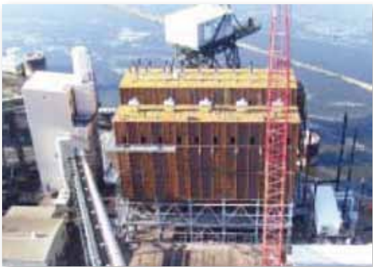
Baghouse construction began at Dairyland Power's Genoa plant in 2007.
