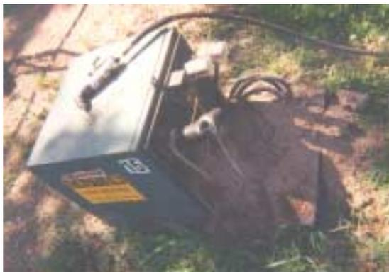
An underground transformer that has had animals living inside of it. Also, the case is rusted and paint is chipping and peeling.
