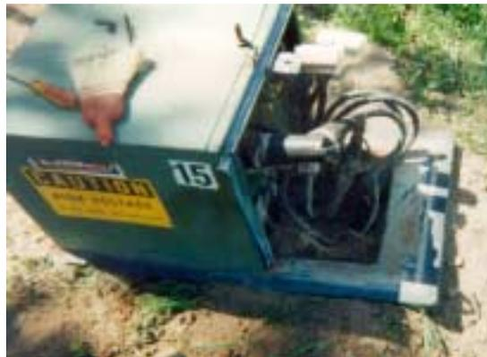
The same transformer cleaned out inside with all the connections tested and in good working order. In the next step the transformer will be repainted and have new stickers applied.
