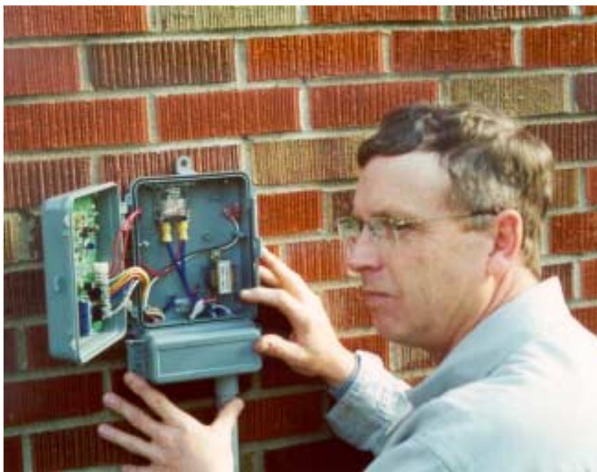
Jim Schemensky, lineman and power-quality specialist, installs a load control receiver on a house. This member will receive \$48/year off his electric bill by allowing this device to be hooked up to their water heater.
