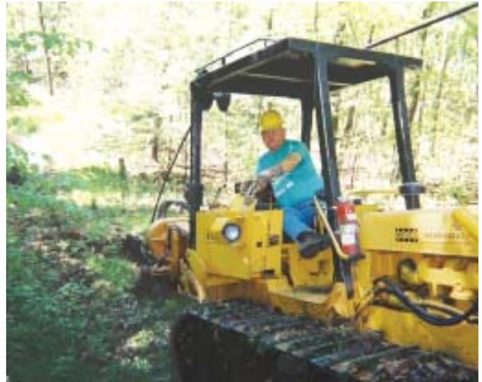
*Equipment Operator Frank Arch plows in the new underground primary conductor in the Chequamegon National Forest.*
