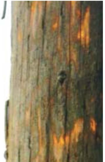
*Here's a pole with its ground cut. This can be a dangerous situation for our linemen and for others during a problem with the electric system.*
