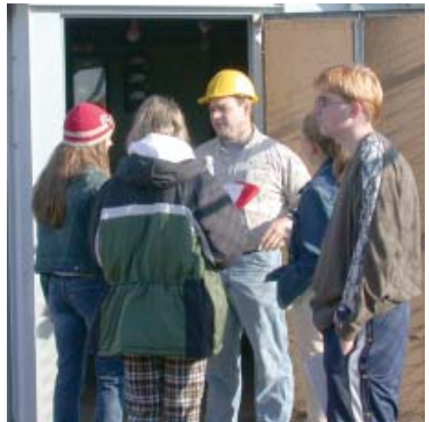
Assistant Line Superintendent Mike Ruff talks to local Greenwood eighth-graders about the controls in a substation.
