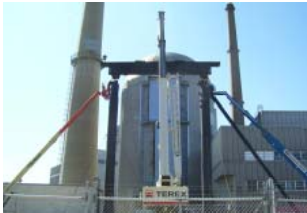
Removal equipment ready to work.
