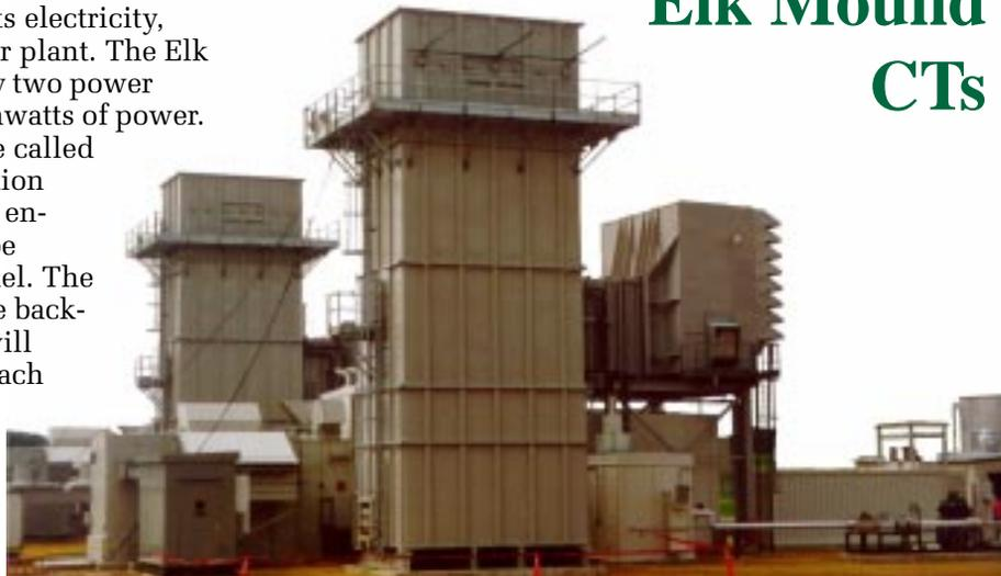
The Elk Mound Power Station—Two combustion turbine (CTs) generators producing a total of 80 megawatts.
